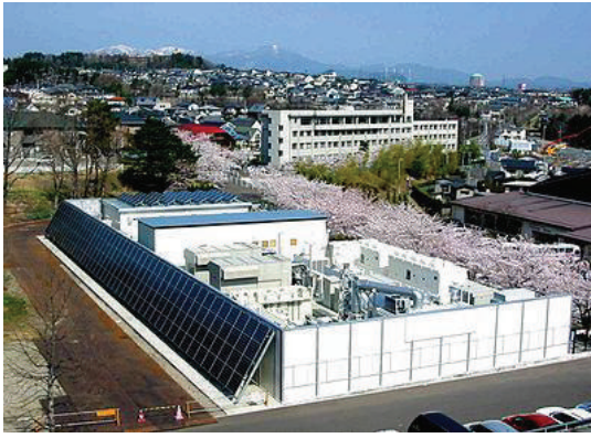
Figure 2: The Sendai microgrid [1], with an output capacity of 1 MW, remained in full service during and after the March 2011 Great East Japan Earthquake, supplying power and heat to the community around Tohoku Fukushi University.
